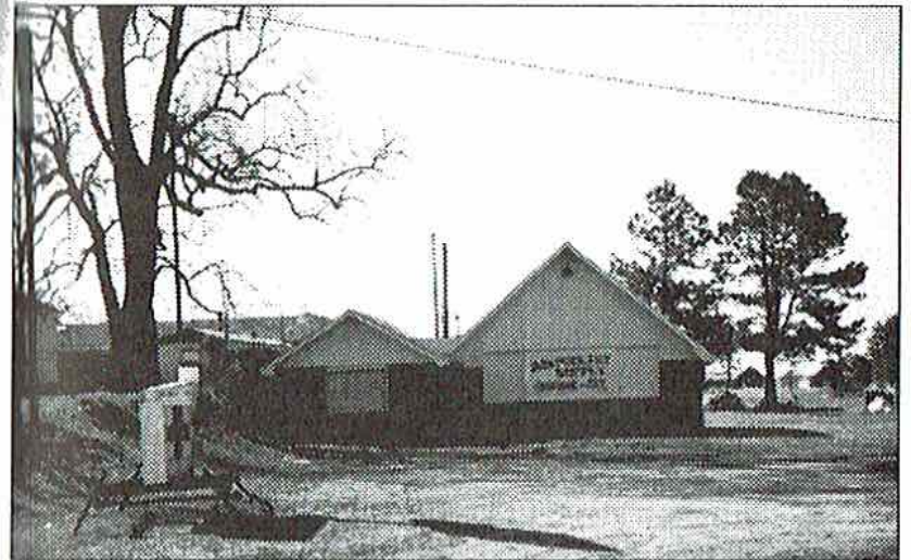
Dutton Poultry Supplies, owned and operated by Winfred Smith was established to service the many poultry growers in the community. Winfred carries chicken houses and poultry accessories.
