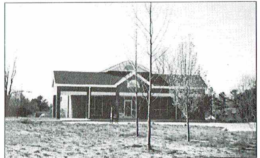
Present Dutton Post Office
